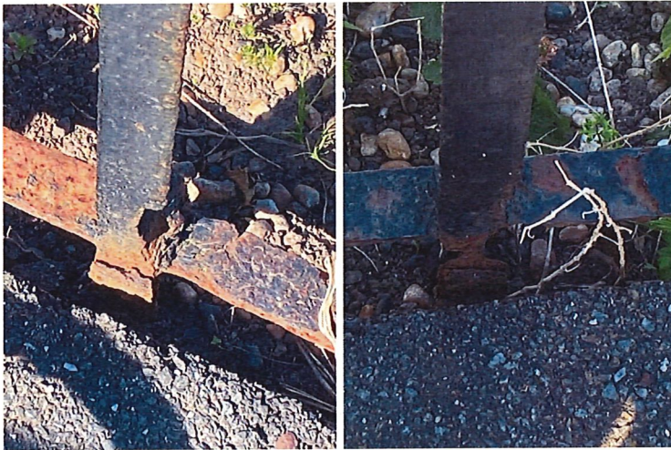
Examples of corroded posts
