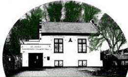
ST. JOHN'S KINGSDOWN VILLAGE HALL
